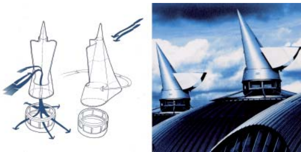
Wind scoops at Bluewater Shopping Centre, Kent, UK
