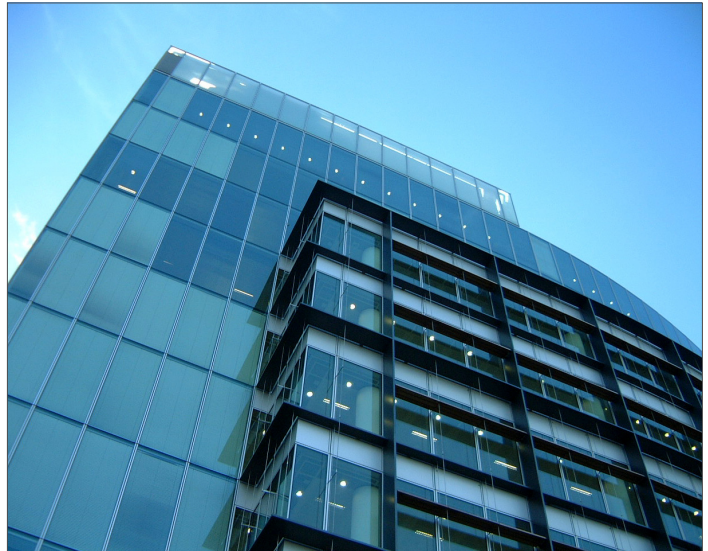
The northern facade of the building. Its conventional cladding conceals a highly sustainable approach to corporate construction
