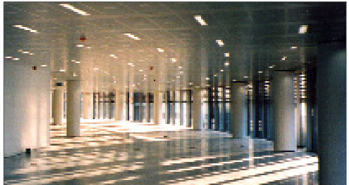
An internal view of the curved structure with full height glazing to allow maximum # penetration of daylight into the space
