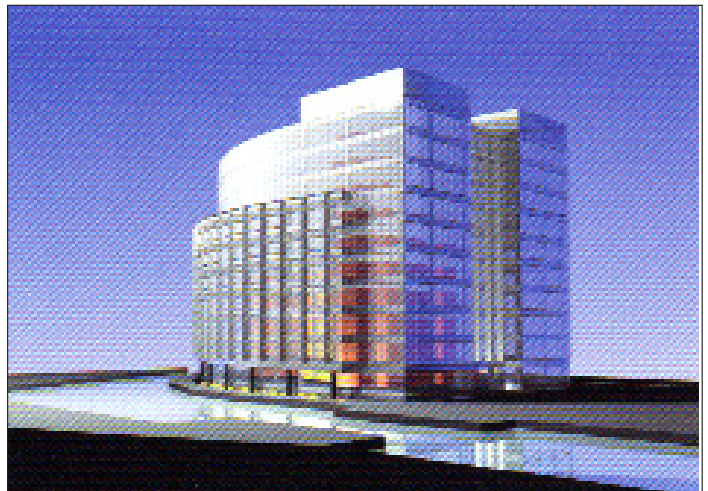
The Point building mass not only responds to the contour of the Grand Union Canal but also reacts to the environment to optimise passive responses.
