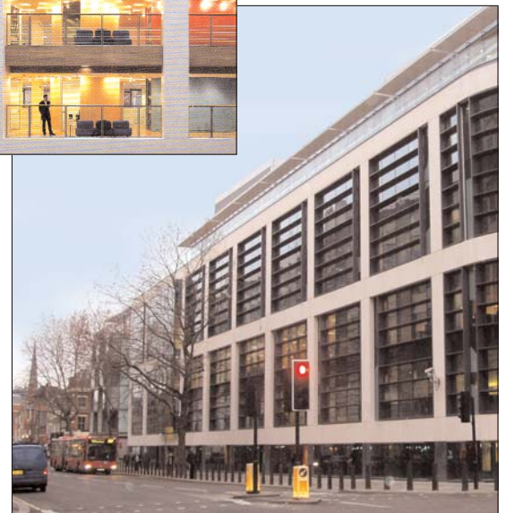
Phased occupation of the buildings began in February 2005
