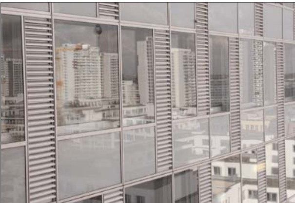
The east facade with silver cladding and aluminium operable louvers
