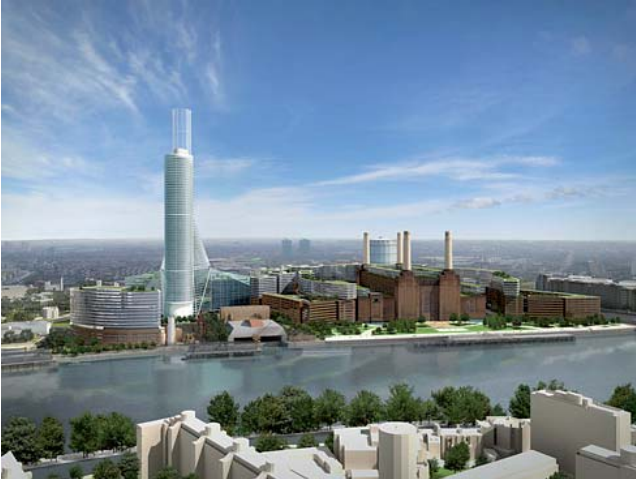
North Embankment View
