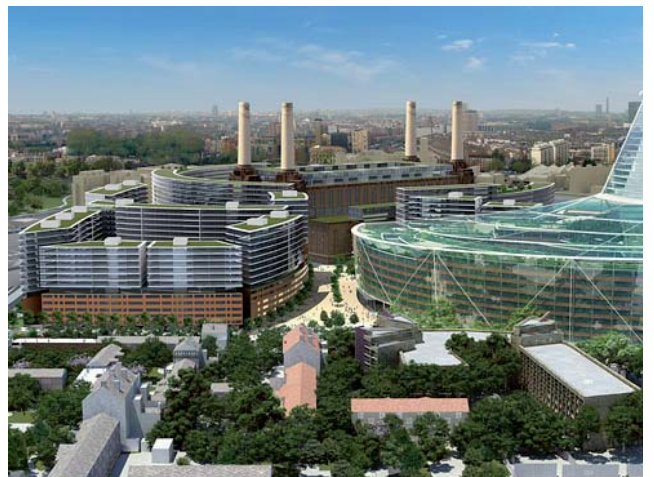
South East view towards Power Station
