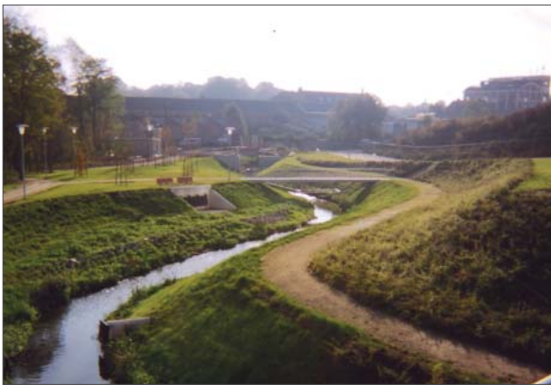
Water management within the landscape
