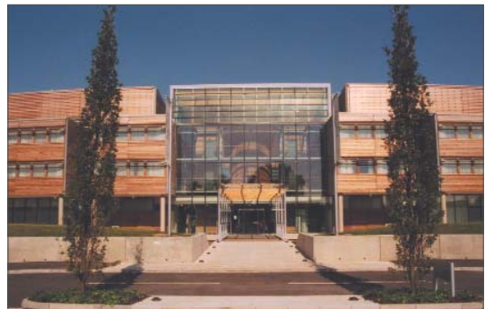
Approach to the main entrance
