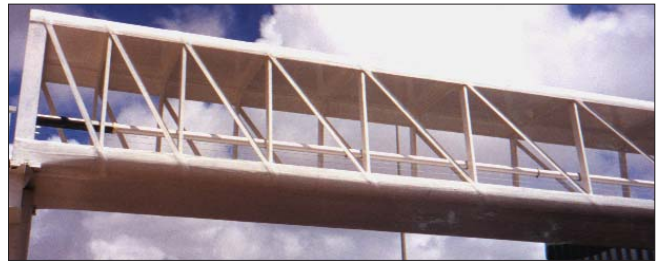
The composite carbon fibre footbridge
