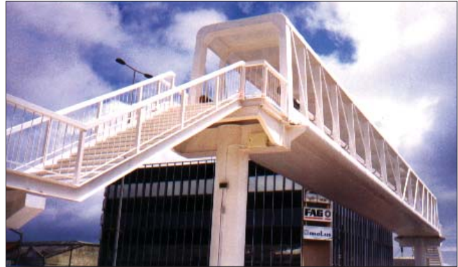
Open sides allow air to circulate
