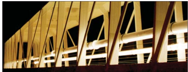
Structural efficiency and design combine to form an elegant urban structure
