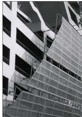
Metal shading devices fit onto the structure on the west facade. These make afternoon work in the offices tolerable.
