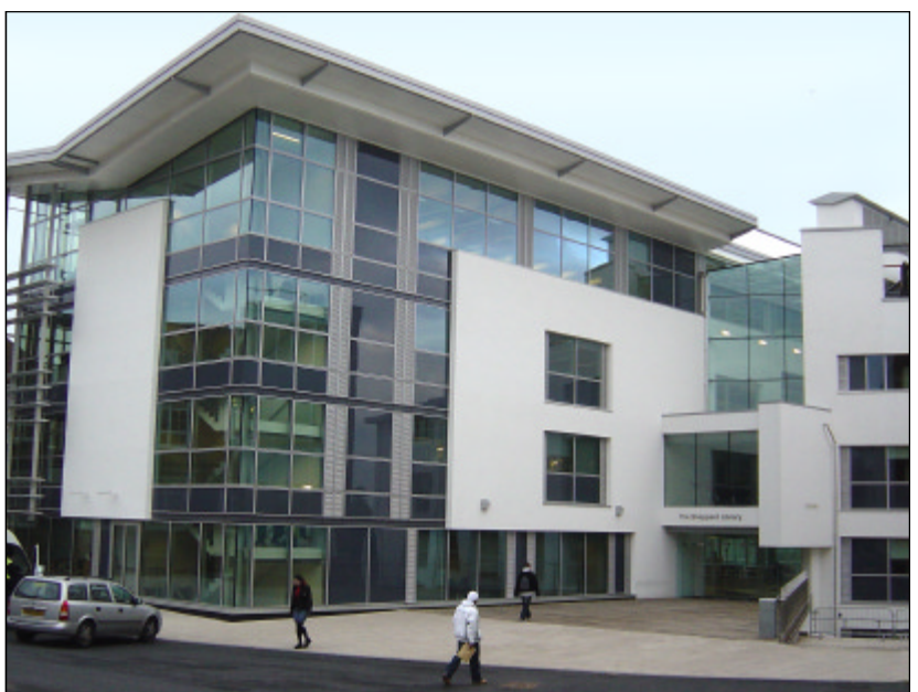
The building in the final stages of fitout - February 2005
