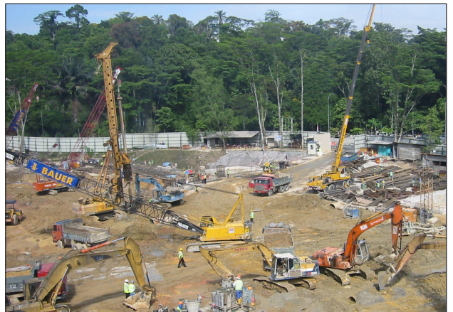
Excavation of the basement storeys began onsite in 2004.
