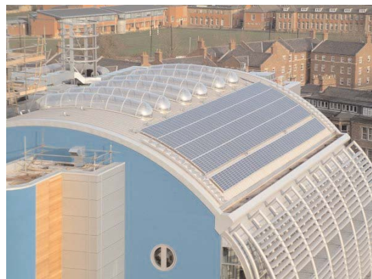
The lightweight roof with PV array, external shading louvers and atrium rooflights
