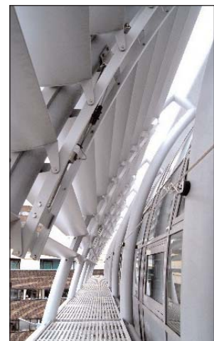
The lightweight roof with PV array, external shading louvers and atrium rooflights
