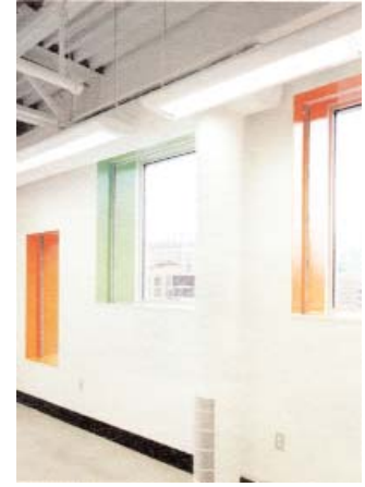
Interior view of brightly coloured window sills
