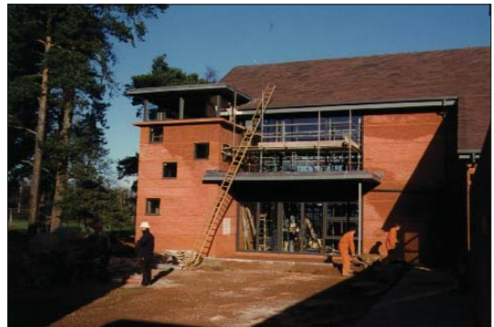
Site Construction Photo's
